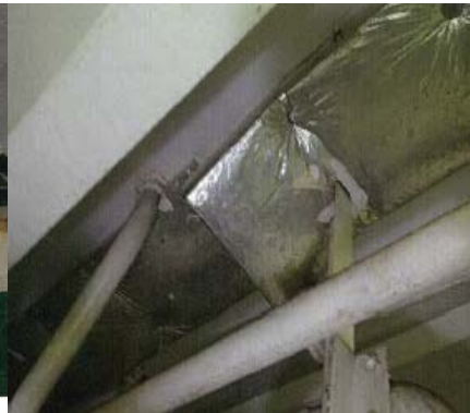
Deteriorated insulation
