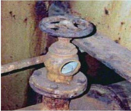
Corroded hydrant and missing coupling
